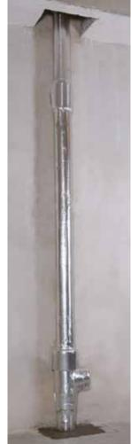
In this simulation, two types of noise level were measured. One was the airborne noise directly in the installation space without further shielding (such as plasterboard) (basement front). The other was the structure-borne noise propagated by the pipe brackets through the installation wall into the room behind it (basement rear). The reference measurement to determine the structure-borne noise attenuation was performed on a sewage system without pipe coating in a mortar-sealed ceiling opening.
